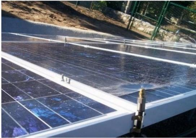
Figure-3. Demonstration of the heliotex method of cleaning solar panels.
