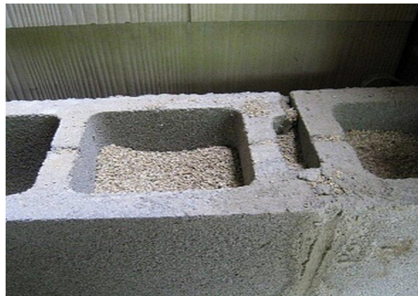
Picture 2. Use of expanded vermiculite in hollow products
