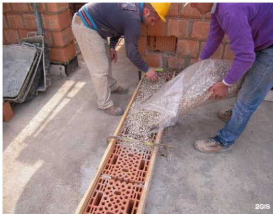
Picture 2. Use of expanded vermiculite in hollow products
